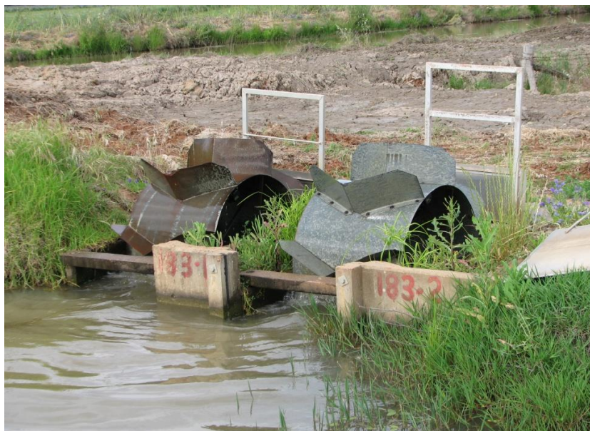
Fig 1.1 Inefficient manually operated Dethridge Wheel meter outlets
