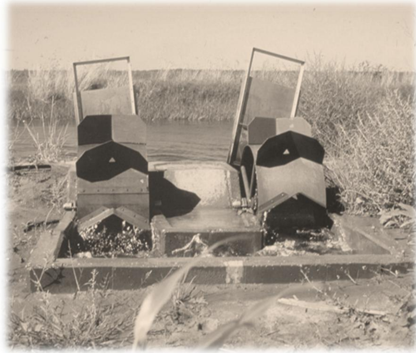
Fig 3.10 Dethridge Wheel meter outlets prior the installation of TCC technology in CIA
