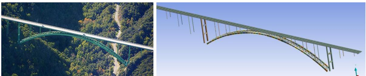
Figure 2: (a) Real Cold Canyon Bridge (b) Finite element model of the bridge
