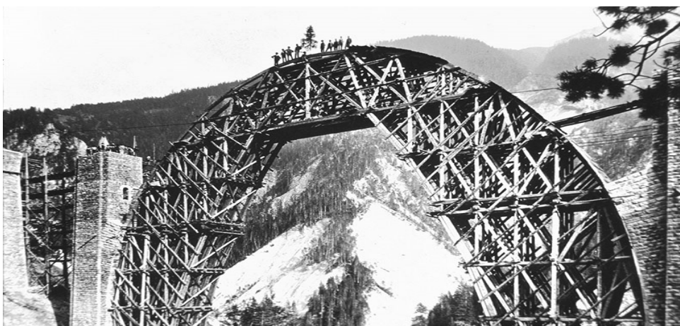
Figure 25: Falsework for bridge
