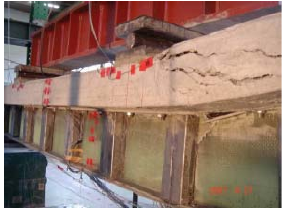
Shear failure of HFRP beam
