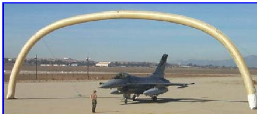
Figure 2.3 Braided air beam by Vertigo Inc (Verge)
