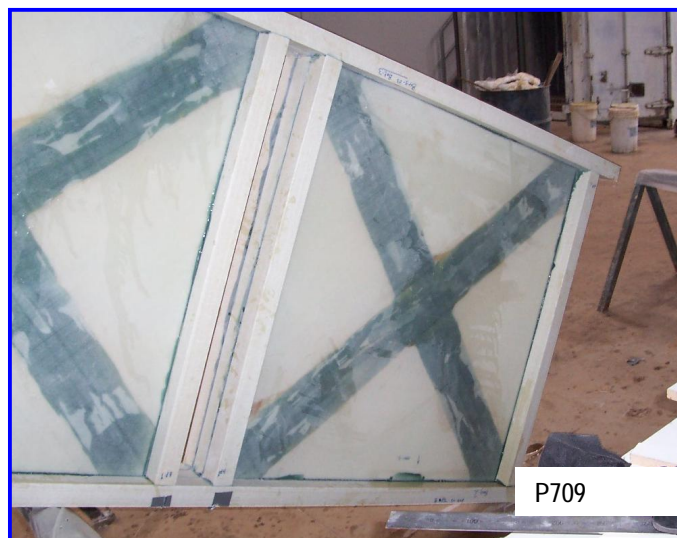
Figure 5.39 P709 - Panel during repair
