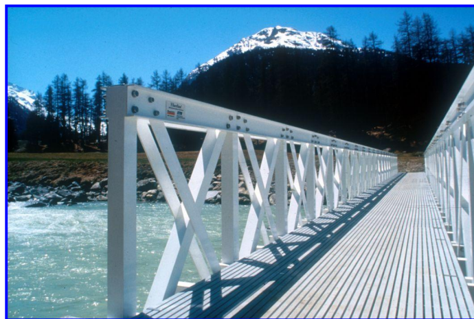
Figure 2.9 Pontresina bridge, Switzerland (Keller, 2001)
