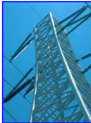
Figure 2.15 Overhead transmission tower using snap-joint ( www.strongwell-ebert.com )
