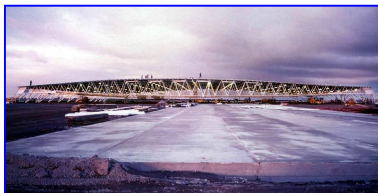
Figure 1.1 Strarch conventional shelters during erection ( www.strarch.com )
