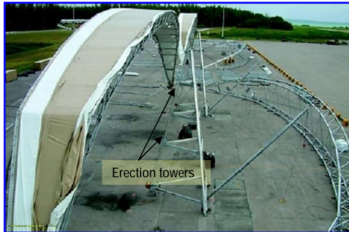
Figure 2.7 XLDAHS Shelter during erection ( www.globalsecurity.org )
