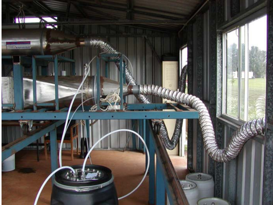
(b) Variable speed fan and odour sampling
