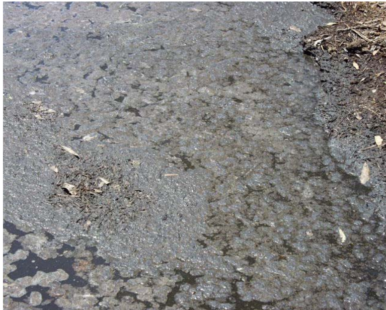
Fig 5.1 Heavily-loaded anaerobic pond with upsurging of sludge
