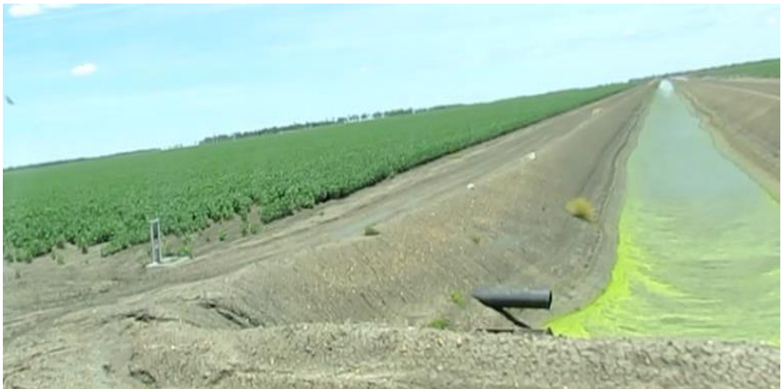
Figure 4.15 Pipe that extends underground from the gated drain box, which is located at the downstream end of the top of Field 2.
