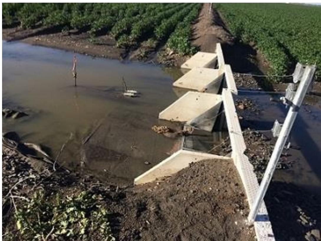
Figure 6.4 Two Starflows mounted on brackets (to avoid mud deposits), downstream of the check gate at the top of Field 2.
