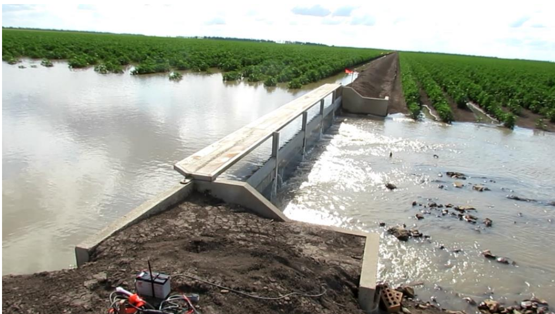
Figure 4.19 An irrigation event in Field 3. This shows the intentional water leakage through the check gate between the metal boards.
