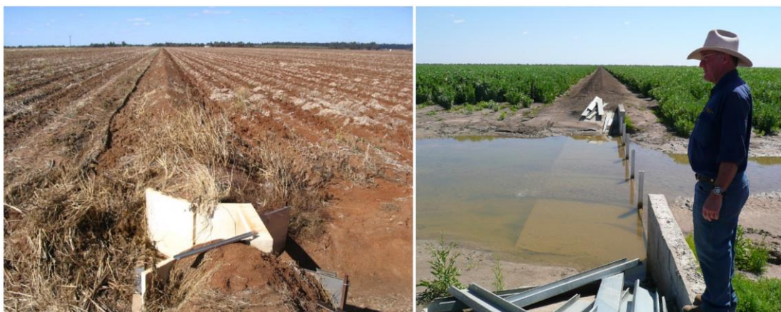
Figure 2.5 Furrowed reverse slope irrigation systems (FRSBO), the left side photo showing an interconnecting (wingwall) culvert between the adjoining borders, while the right side photo showing an interconnecting check gate between the adjoining borders.
