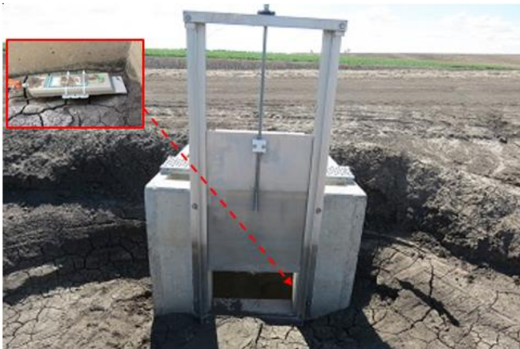
Figure 6.6 Starflow mounted on a bracket inside the concrete structure of the head drain box top of Field 2.
