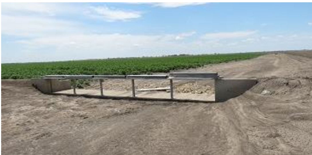
Figure 4.10 Check gate at the top of Field 3
