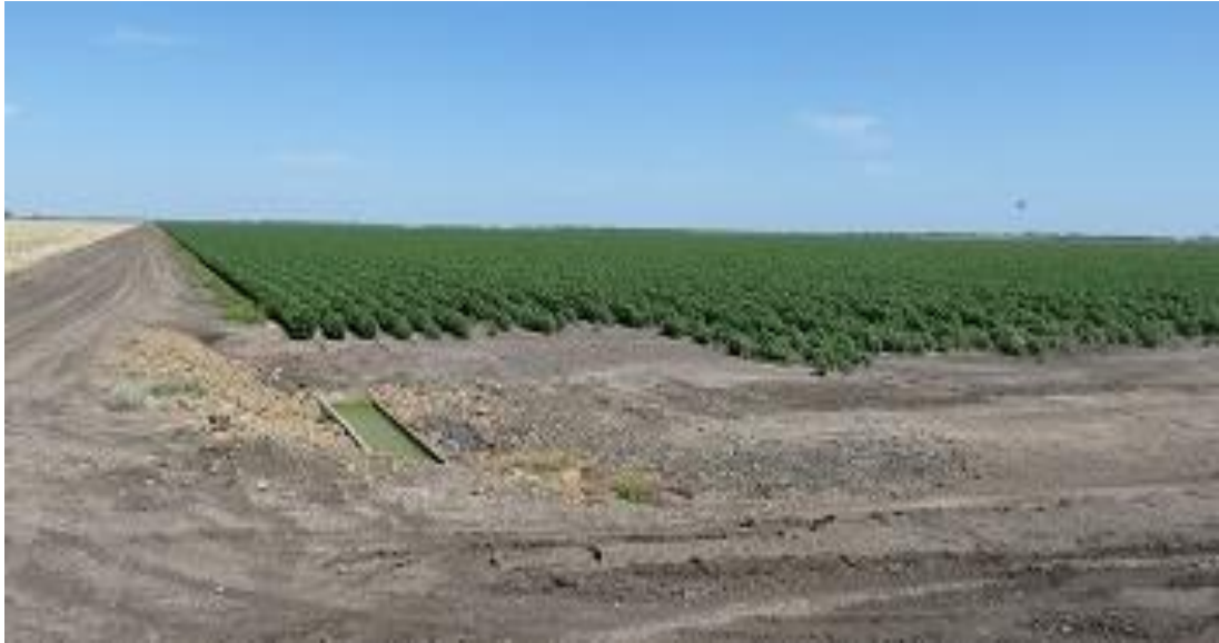
Figure 4.13 Inlet structure at Field 3
