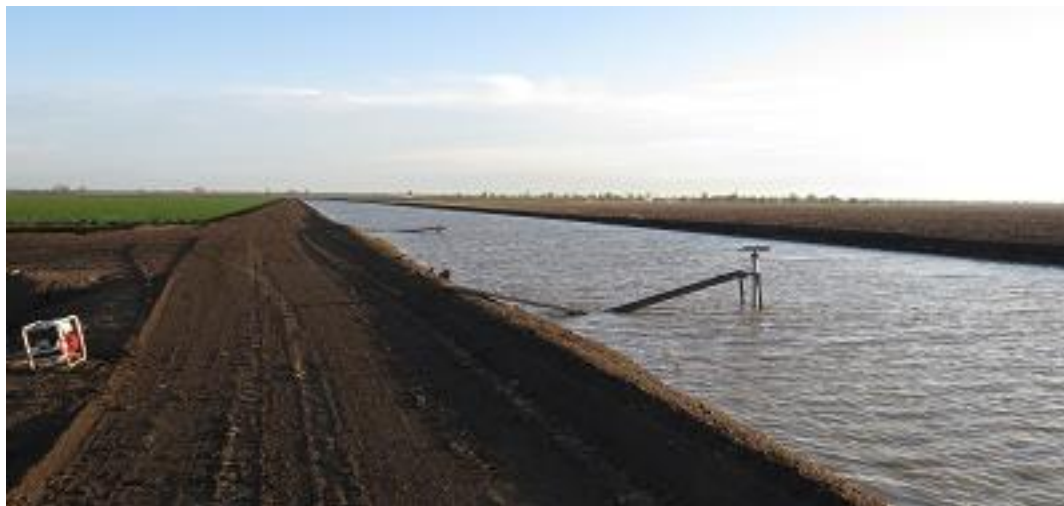
Figure 4.8 Knife gate at the top of Field 2 (includes walk way and hand wheel mounted in the main channel) that feed from the main channel to the water supply inlet, during the irrigation event.
