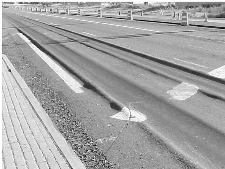
Figure 1.1: Severe creep deformation on flexible pavement (Pavement interactive 2012)
