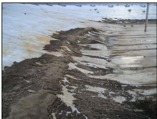
Figure 5-33 Silt and wind blown debris have the potential to stretch the cover and allow water to sit on top of the cover. Silt and debris should be removed, without damage to the cover, while the water level is low to allow the cover to float as the water level rises.
