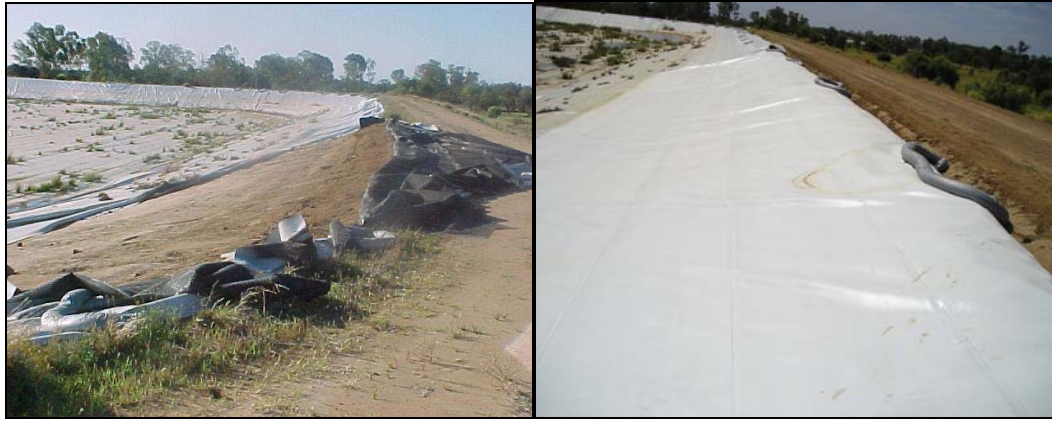
Figure 5-30 Tears should be addressed immediately by sand bagging the torn edges and contacting the installer to arrange repairs. Damage done to this cover was repaired as soon as possible after the tear to limit further damage and maintain effectiveness of the cover. The photo on the right shows the cover after the repairs had been done.
