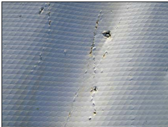
Figure 5-31 Minor damage caused by animals may initiate large tears in the cover.
