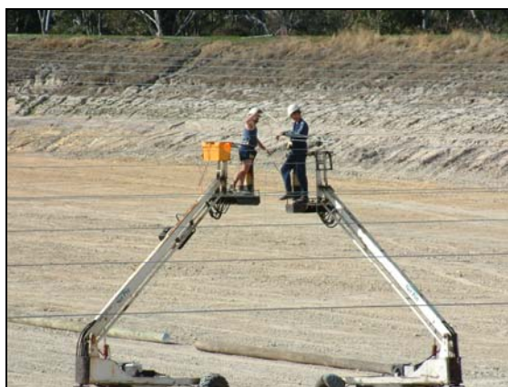
Figure 5-35 Installation of the high tension cables which are anchored into the wall of the storage.
