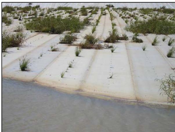
Figure 5-11 The E-VapCap cover with weeds growing out of the drainage holes and restricting drainage of rain off the cover. Weeds from seeds blown onto the cover during dust storms should be dealt with at the earliest opportunity after germination, with a low strength spray application. No other covered storages have reported such problems.
