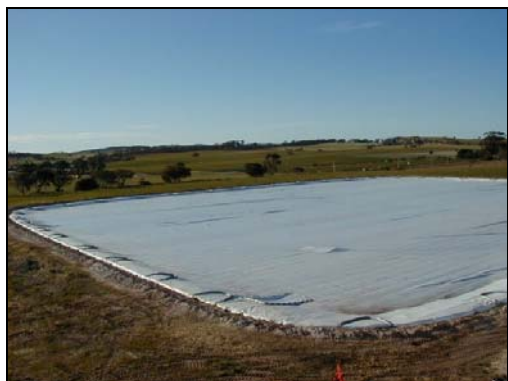
Figure 5-34 The 1.3ha storage in the Barossa Valley, SA had a removable panel installed to service a floating pump.
