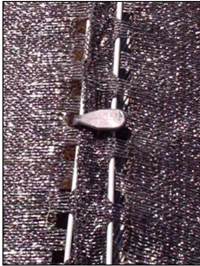
Figure 5-36 The seams in the shade cloth are joined by wires and clips. Any damage to the seams should be repaired as soon as possible to avoid even further damage.
