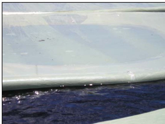
Figure 5-16 Water pooling on top of the Raftex modules after rain or wind events.
