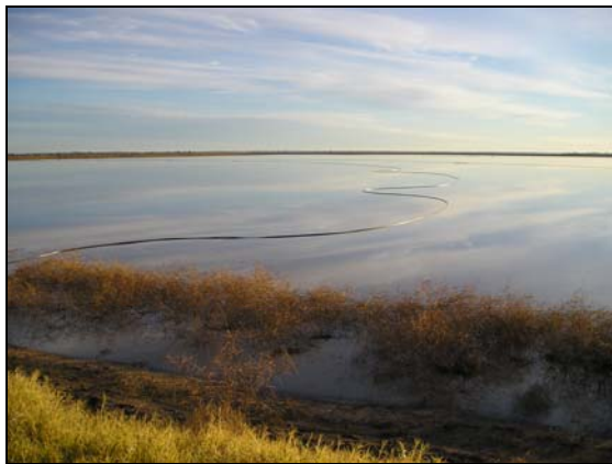
Figure 5-25 The polythene pipe floating on the water surface would pull apart at the joints or break the rope that was used to tie in place. This problem can be overcome by burying the pipe underground.
