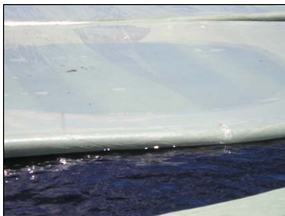
Figure 5-40 Water sitting on the modules gets there by rain or by the wind blowing and waves going over the edge. The water does not drain off here and will only evaporate.
