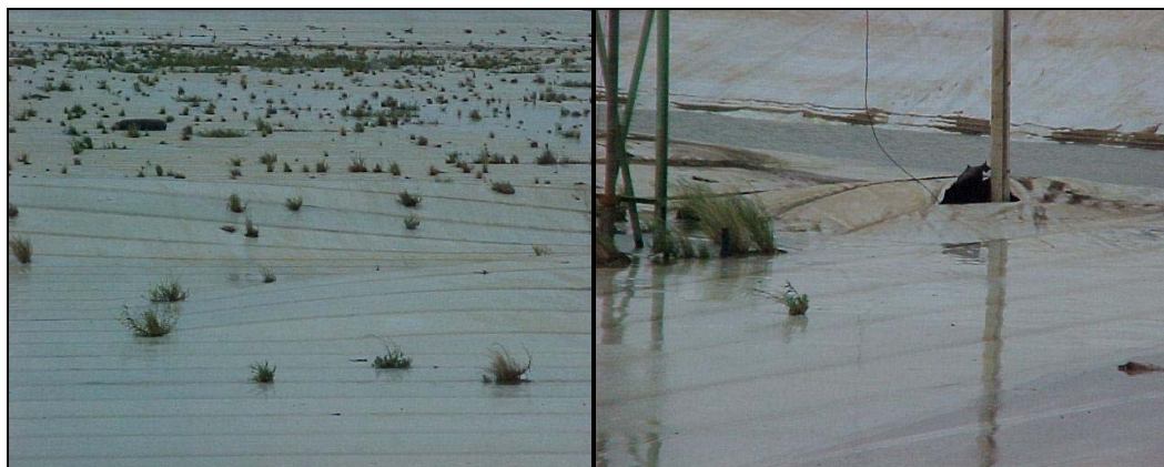
Figure 5-29 Wind under the cover has the potential to make small tears larger and ‘pump’ water on top of the cover. Any subsequent addition to structures after completion of cover should be in consultation with the installer.
