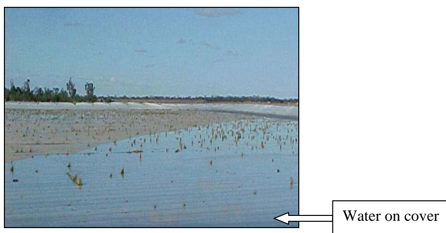
Figure 5-9 Thin layer of water may cover a large area of the E-Vap-Cap after rain or strong wind event. This should drain through the cover into the storage after the wind or rain ceases.
