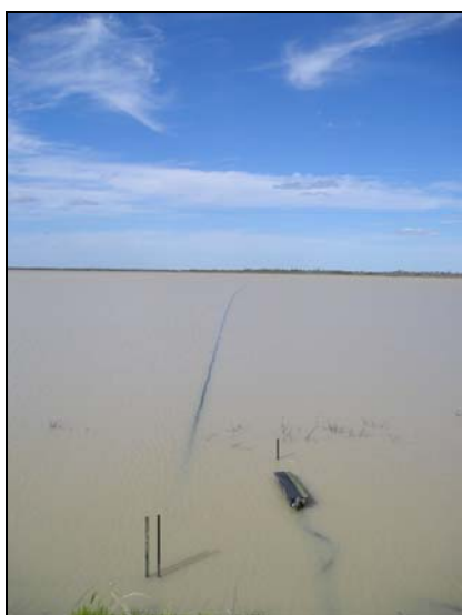
Figure 4-19 The polythene pipe floats on the surface of the water and is tied at either end to hold the outlet points in the right position. Ideally the pipe should be placed on the floor of the storage as the wind and waves affect the pipe grid system.
