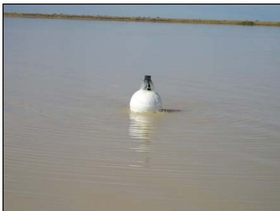
Figure 4-18 Nine outlets are evenly spaced across the 120ha storage. The main distribution lines are 50mm polythene pipe and then each riser has 10-20m of flexible hose with its own float system.
