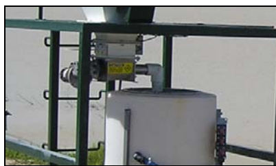
Figure 4-15 Water$avr powder is metered out of the hopper using a screw auger.
