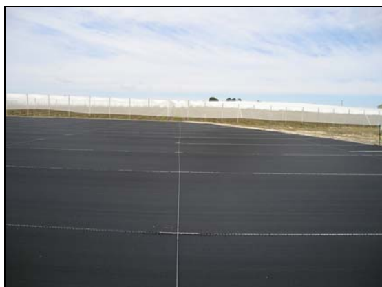
Figure 3-10 NetPro shade cloth structure over a 3.8ha storage at Stanthorpe showing orchard with hail protection on two sides of the storage.
