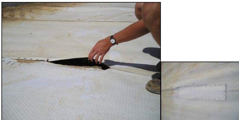
Figure 5-32 Damage to welded seams should be repaired as soon as possible. The tear can become much larger if wind is allowed to blow under the cover.
