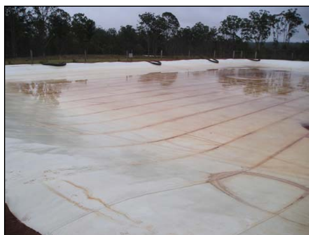
Figure 5-10 A 0.28ha storage at Hampton during a rain event showing thin layer of water on the surface which drains through the drain holes once the rain ceases.
