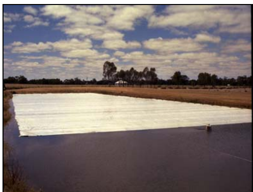
Figure 5-26 The 0.25ha E-VapCap product covers 60% of the surface area of the storage at Quantong, Victoria at the client's request and uses a tethered method rather than the trenched method.
