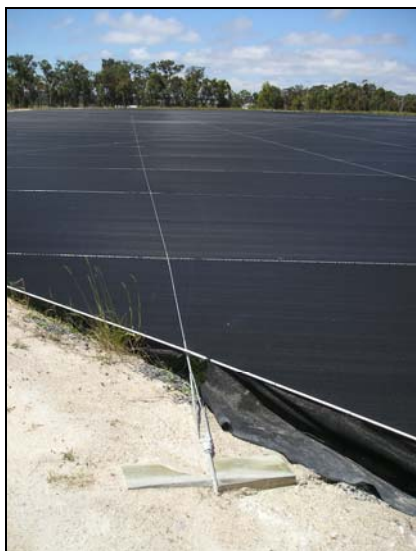
Figure 5-38 Around the perimeter of the main shade cloth structure is a curtain that hangs over the edge of the to reduce the amount of wind getting under the cover but still allow any silt that is eroded off the storage bank not to sit on top of the cover.
