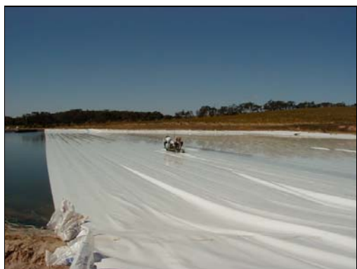
Figure 5-27 Welding of the seams during installation on a 1.3ha storage in the Barossa Valley, South Australia.
