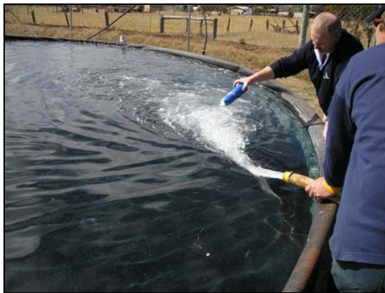
Figure 5-43 Application of PAM requires the contents of the storage to be completely mixed.
