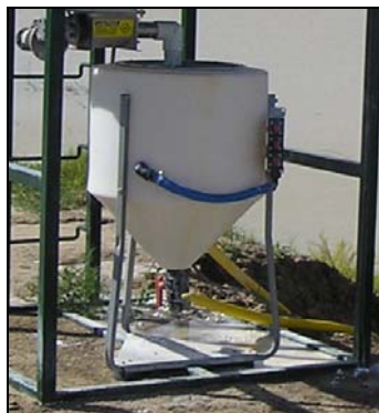
Figure 4-16 Dry powder is mixed with water from the storage in the mixing chamber.
