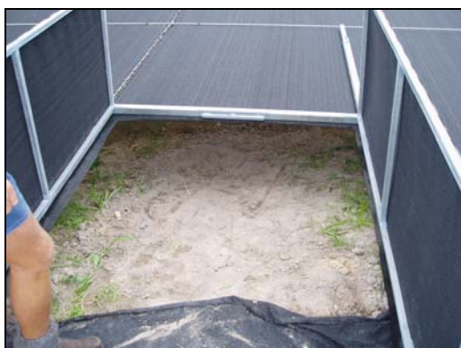
Figure 5-39 A gateway entrance was retrofitted to the cover to allow access under the cover.
