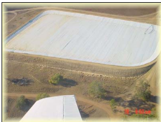
Figure 3-9 The E-VapCap cover just after it had been installed on a 4.2ha water storage at St George.
