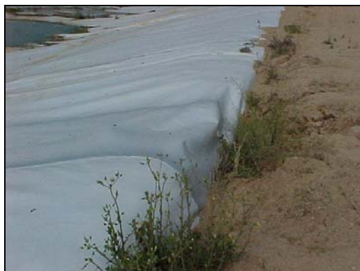
Figure 5-28 The anchor point along the bank used in the trenched system is susceptible to erosion especially if the bank is graded inwards. Alternatively, a gutter with drains can eliminate this potential problem.
