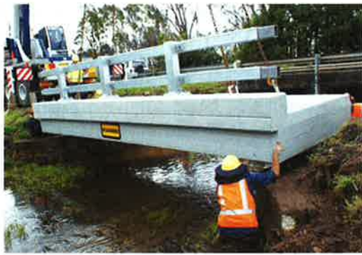
(a) Manly Road Bridge ( www.wagnerscft.com.au )
