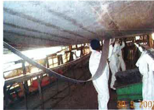
(b) Structural strengthening of West Gate Bridge [12]
