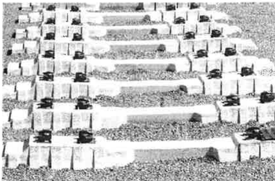
(a) Sleeper made of polymer concrete and fibre composites
