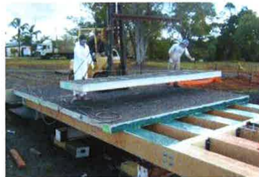
(b) New generation composite bridge at USQ
