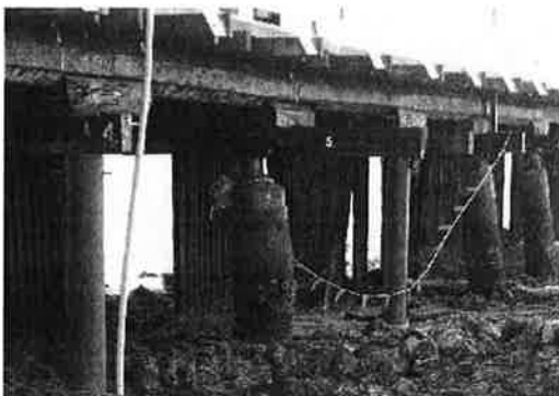
(a) Timber pile replacement at Shorncliffe pier
