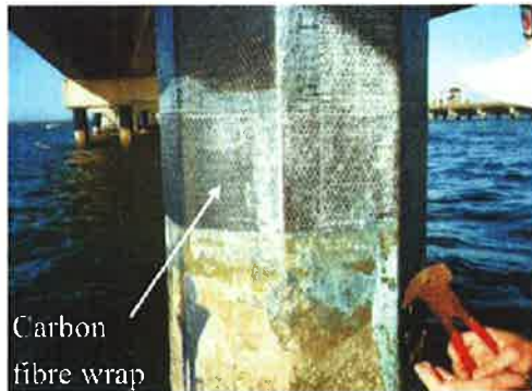
a) Repair of pre-stressed concrete piles
