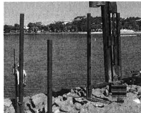
(b) Composite piles for Jack Evans Boardwalk
