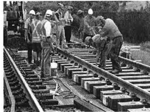
(b) Fibre composite transoms
