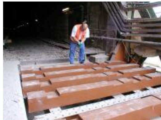
(b) Railway track in Zollamt Bridge
