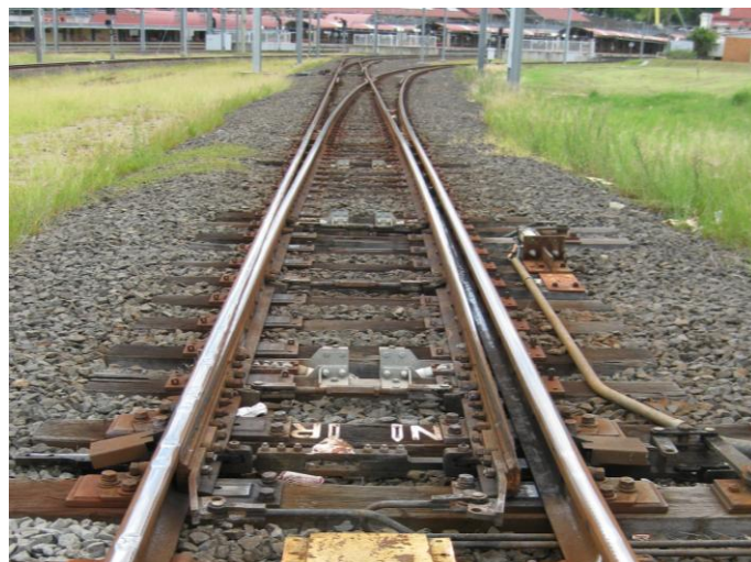
Figure 1.2 Right-hand railway turnout structure
