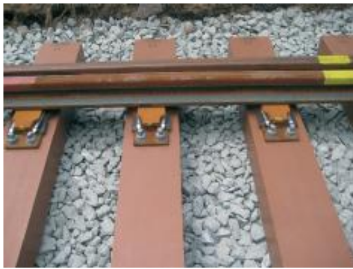
(a) Mainline railway track
