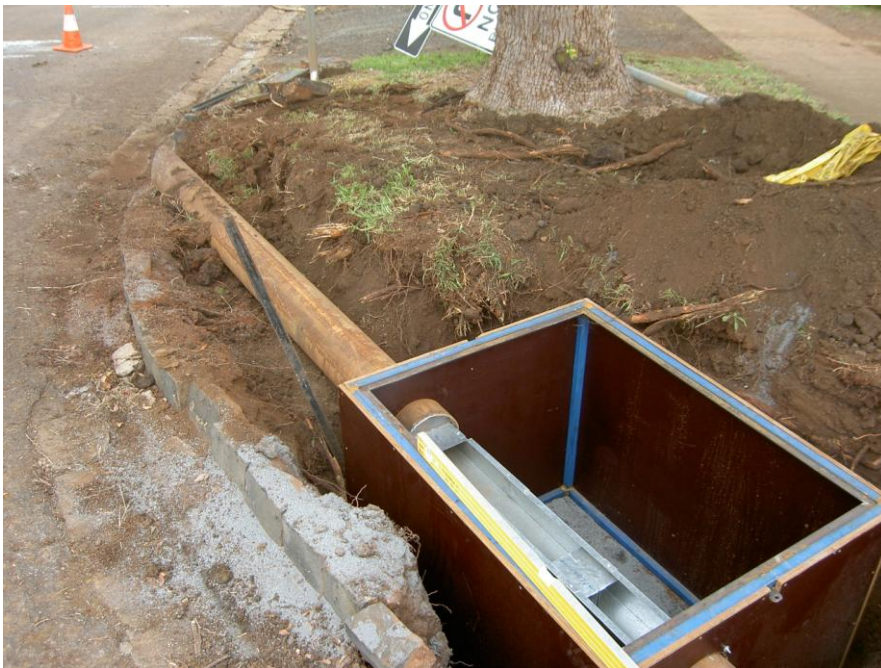
■ Figure 6.10 Photograph of the road sampler being installed
