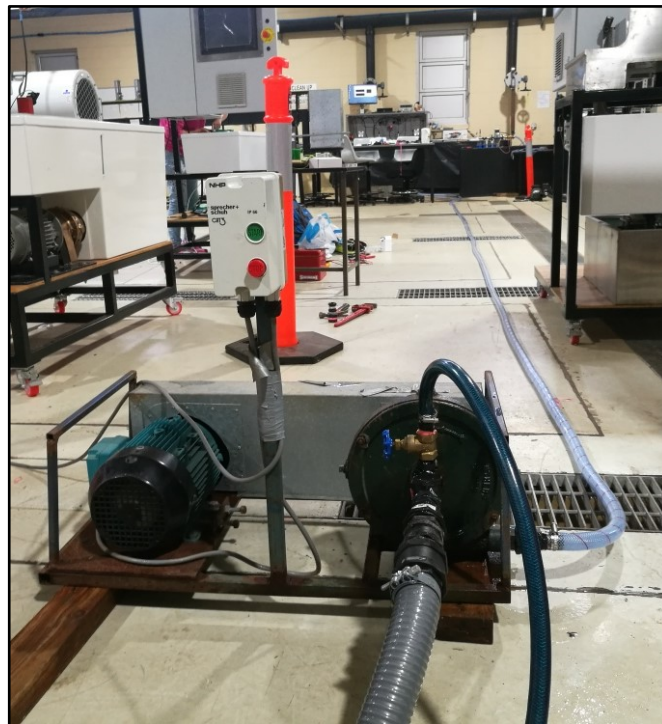
Figure 4-8: Southern Cross pump connected and running from underground storage tank
